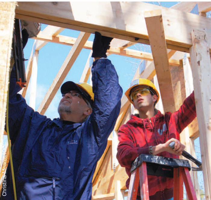
Father Dimitrios Antokas and a young volunteer work side by side to help secure the framing on this storm-damaged home. More than 100 Orthodox faithful volunteered their time to IOCC Action teams this summer to restore homes and hope to families who lost everything to natural disasters.
