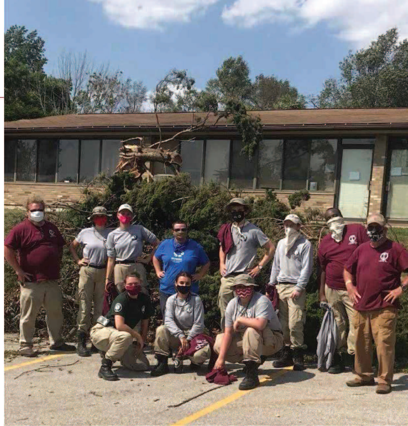
IOCC lead a team in Cedar Rapids (above) following destructive windstorms, including clearing fallen trees from yards and driveways (below left).
