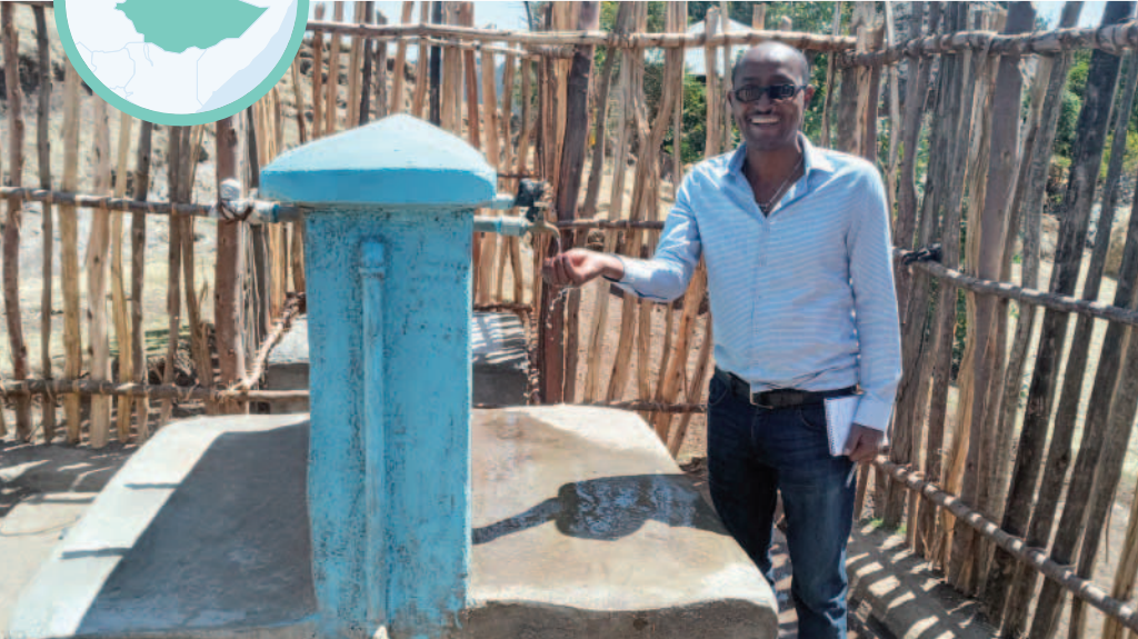
This spring in Ethiopia is now covered so the water will stay clean, and people can use the faucet to fill their containers.
