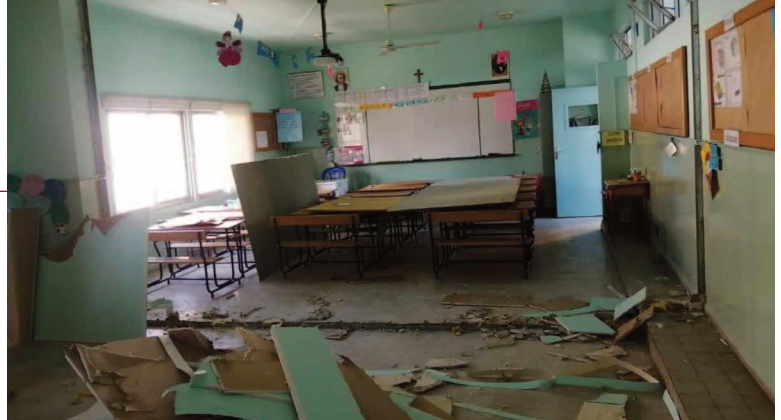
Two classrooms, shown here with their partition wall that the explosion destroyed. Image continued from cover below shows the same space repaired.
