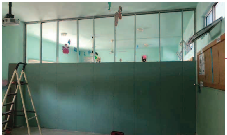
Repairs facilitated by IOCC replaced the wall between these classrooms — one small example of the past year's rebuilding efforts.
