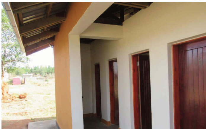
A new central sanitary block ensures that students at this rural Ugandan boarding school have a safe, healthful learning environment.
