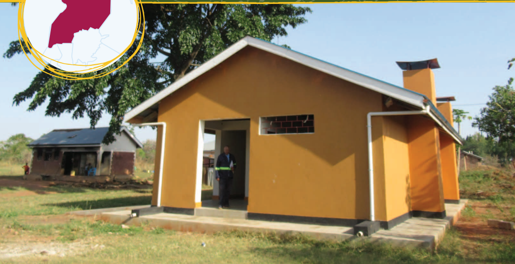
A new central sanitary block ensures that students at this rural Ugandan boarding school have a safe and clean learning environment.
